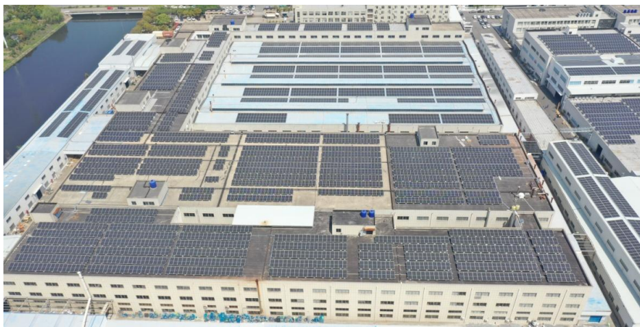
Fig.5 Quzhou Shanshan new material cement rooftop project
